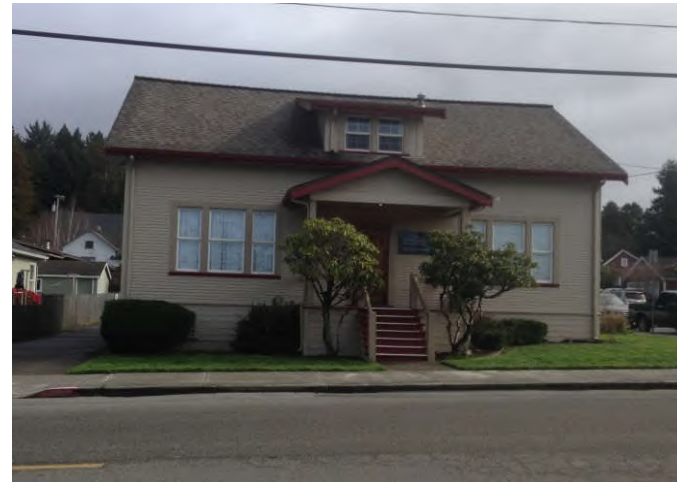
Photograph 4. Church located at the intersection of 13 th and B Streets, facing east
