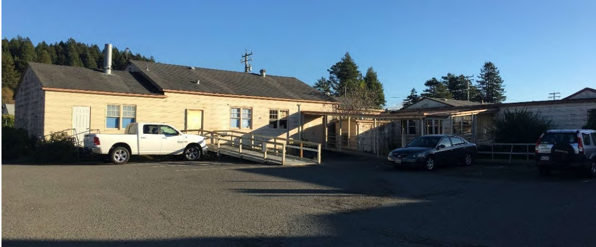
Figure 13 West Elevation of Former Laundry/Boiler Room with Connecting Breezeway
