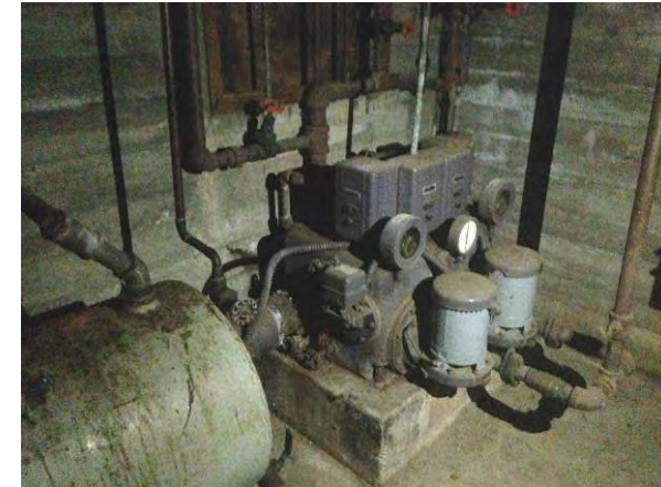
Photograph 6. View inside of the basement boiler room.
