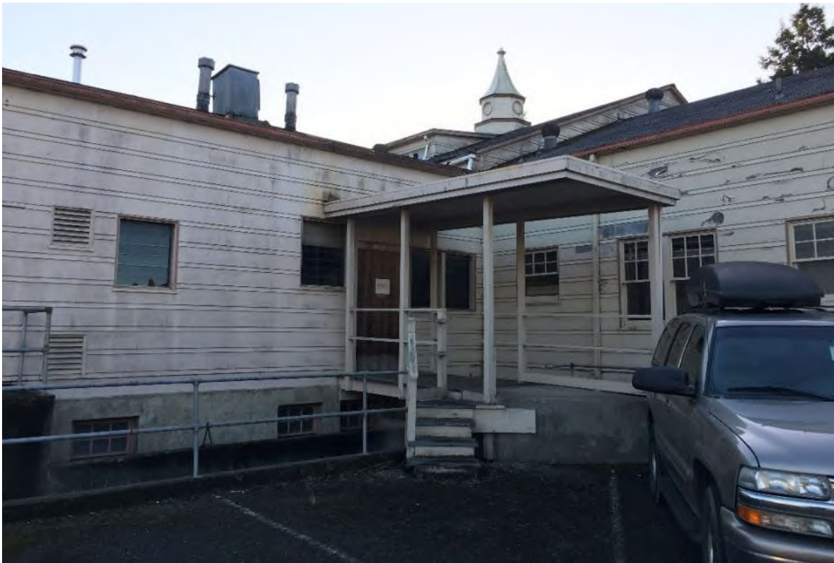
Figure 14 Entrance at Northeast Portion of North Wing, Looking Southwest
