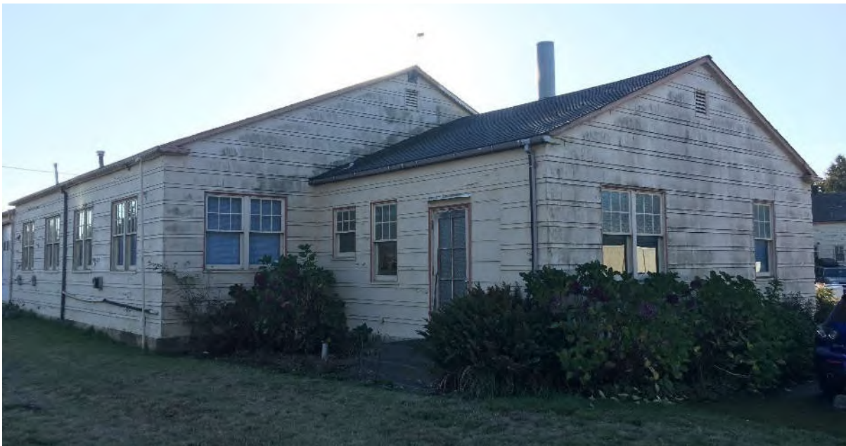
Figure 12 Main Block, Boiler Room and Laundry
