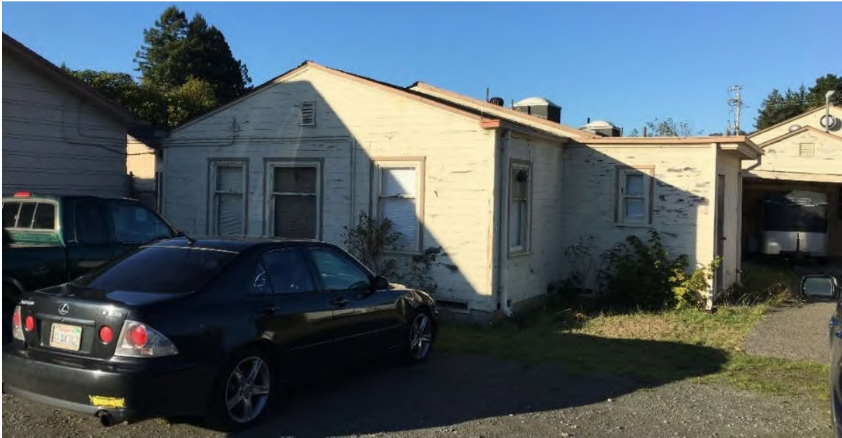
Figure 11 Main Block, Sisters' Quarters
