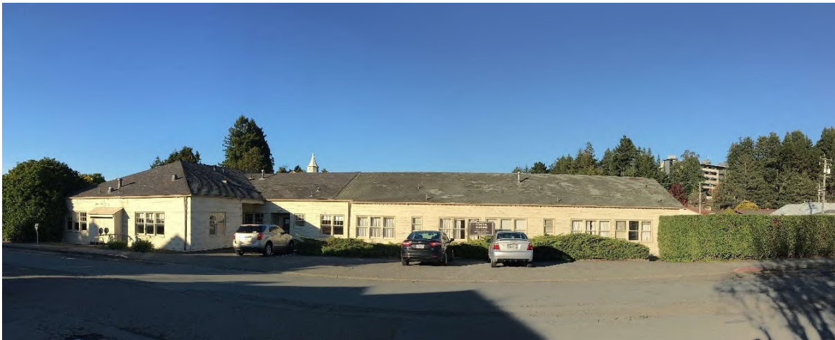
Figure 16 Overview of 1956 Extension (Left) and 1948 Addition (Right)
