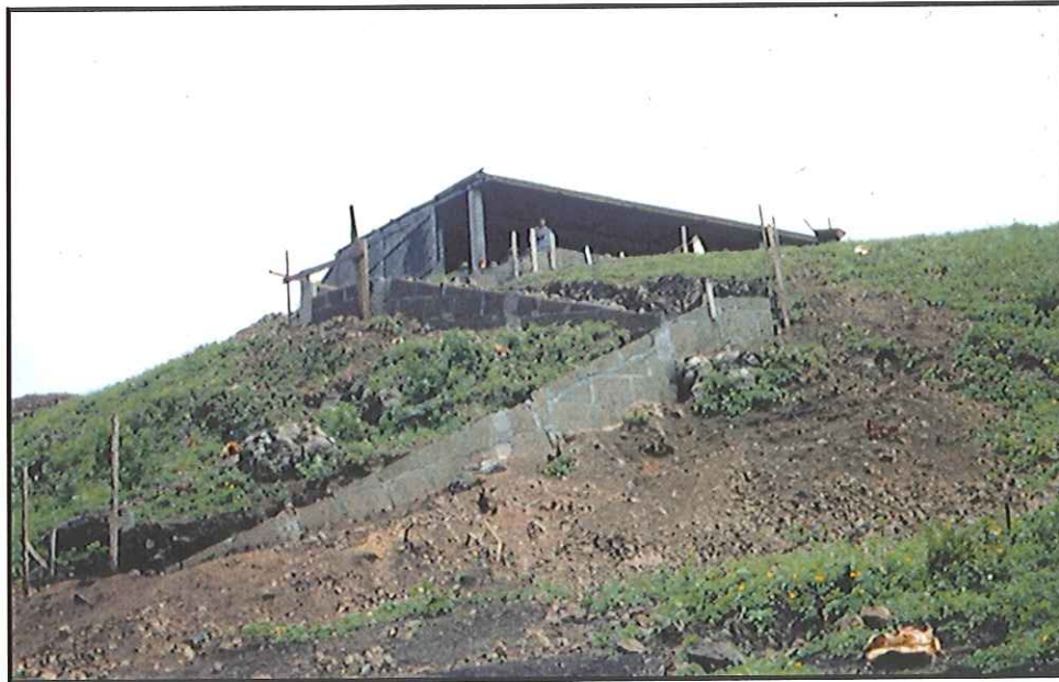
Project Site After
