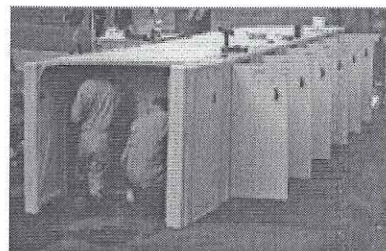
Installing bicycle lockers
