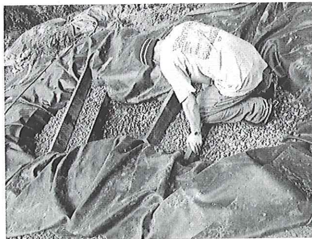
Figure 5 Redwood baffles being adjusted after gravel was shoveled in
