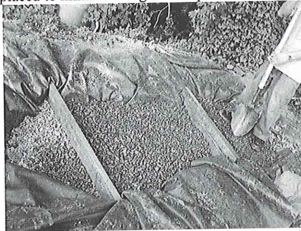
Figure 7 Gravel being shoveled into marsh prior to planting
